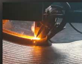
Pressure Vessel Cladding
