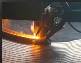
Pressure Vessel Cladding
